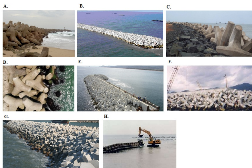
Figure 3. Breakwaters made of prefabricates of various types: (A) Dolosse, (B) Accropode, (C) KOLOS, (D) Tetrapod, (E) Core-loc, (F) A-Jack, (G) Xbloc, (H) Waveblock [19].
